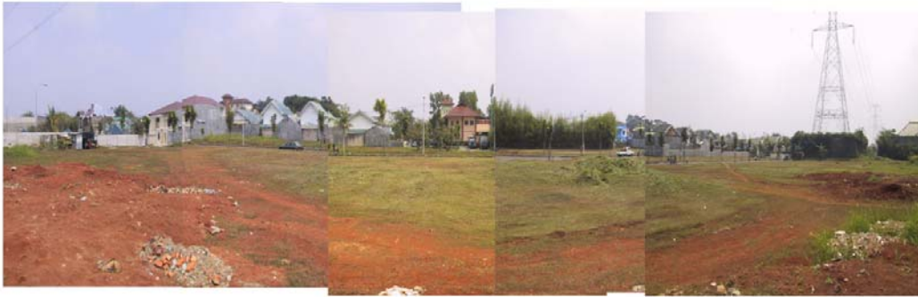
A panoramic view of the site. (photo by Adi Purnomo)
