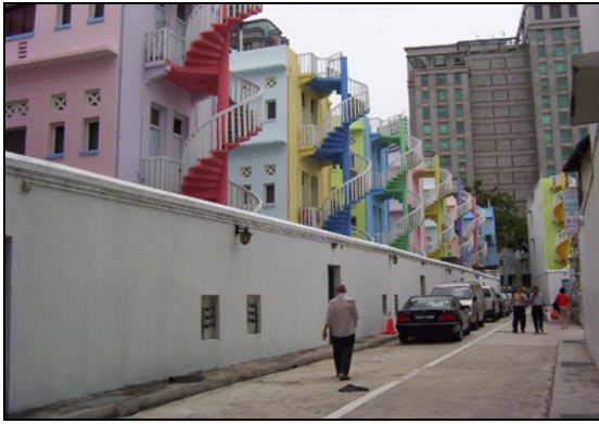
Backside of buildings, Bugis Village- Singapore (Photo by. Fransiska)
