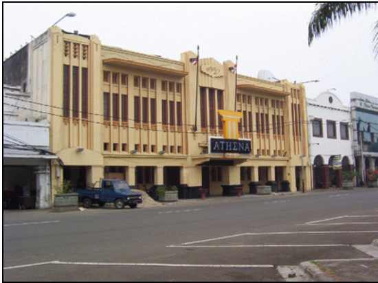
Athena-yellow colored- as an attempt to infill new color in Jakarta Kota's famed Kali Besar warehouse area.
