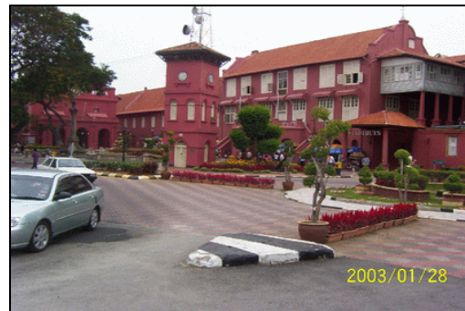
Stadhuys-Malacca, built between 1641-1660 The Malacca municipal Council painted the historic buildings all Red though is not the original color historically. (Photo by. Fransiska)
